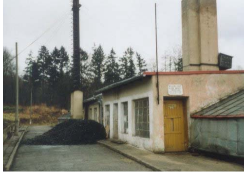
Figure 6.18 The boiler house in Jelenia Góra
