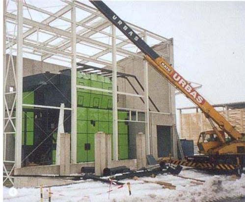
Figure 6.6 Assembly of the biomass plant
