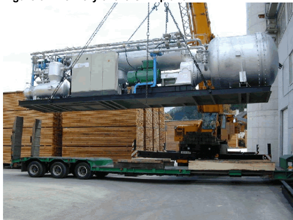
Figure 6.4 Delivery of the ORC plant
