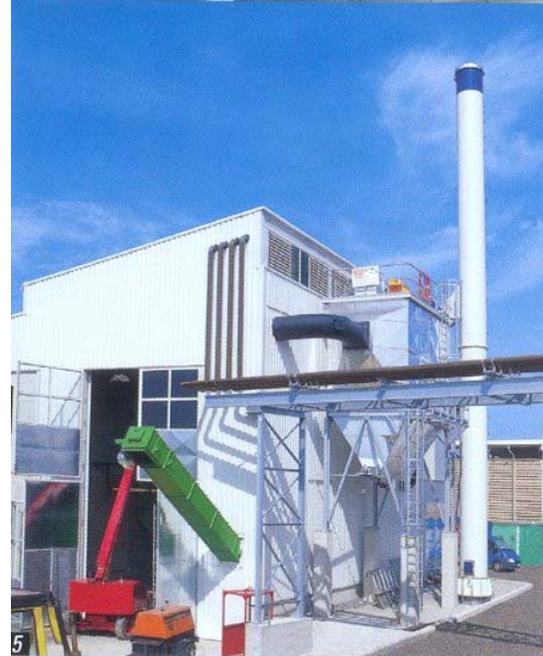
Figure 6.7 Completed biomass plant
