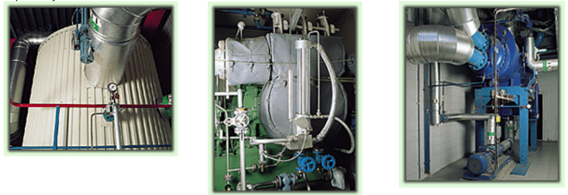
Figure 6.17 Equipment after erection: flash-box, turbine with generator and vacuum condenser respectively
