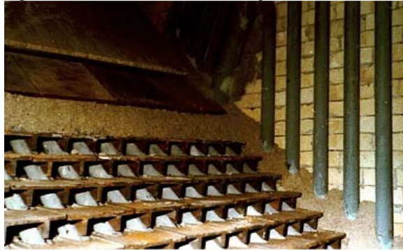
Figure 3.7 Picture of an inclined fixed grate
