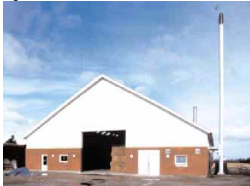
Figure 6.8 The boiler house in Søndre Nisum
