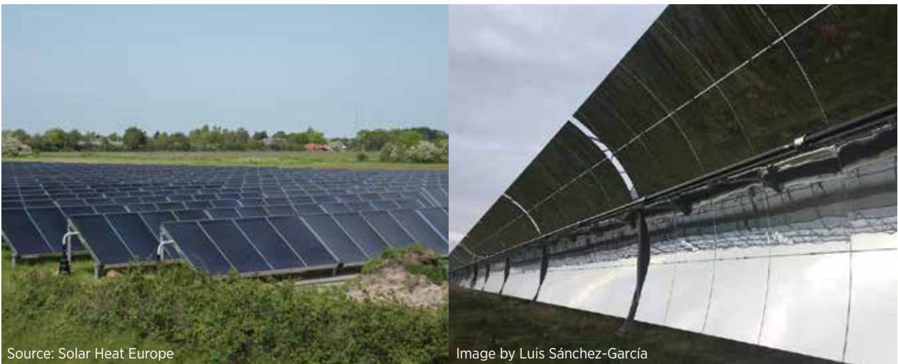
Photograph 2. Solar plants with flat-plate collectors in Løgumkloster (Denmark) (left) and parabolic trough CSP in Brønderslev (Denmark) (right)
